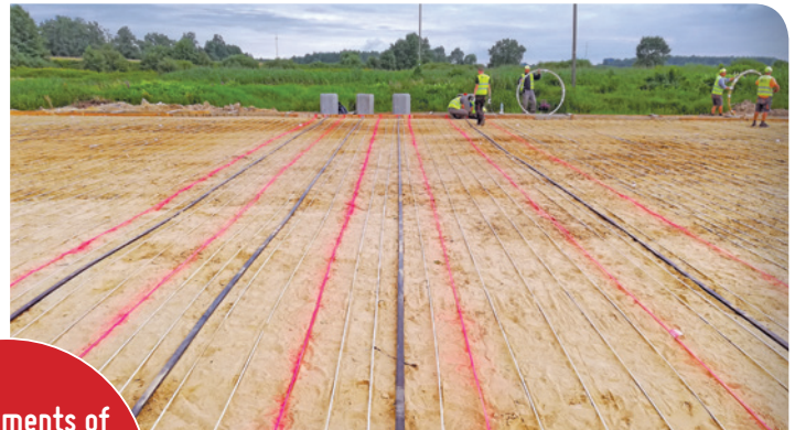
Application of 3DSensor in a road embankment
