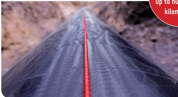
Application of EpsilonRebar on a steel gas pipeline
