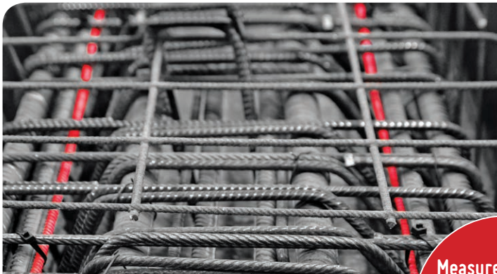
Prestressed concrete beam with EpsilonRebar
