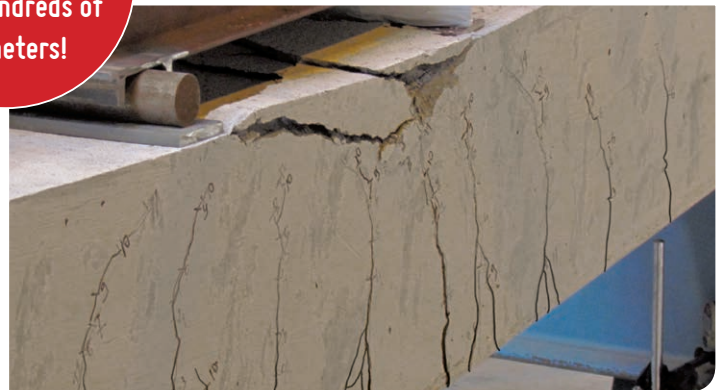
Crack measurements by EpsilonSensor during bending tests
