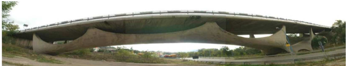
Fig. 2. View of the reinforced concrete bridge erected in 1969 (Potenza, Italy), monitored using distributed fibre optics [8].
