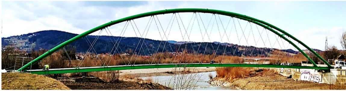
Fig. 6. View of the finished pedestrian-cyclist footbridge in Nowy Sącz.
