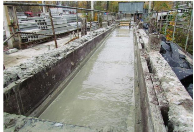
Figure 10. The view of smart girder just after concreting
