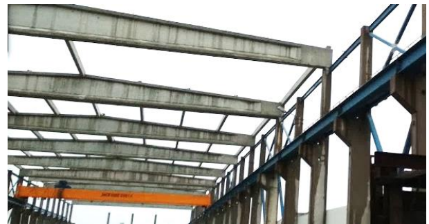
Figure 15. The view of smart girders during construction stage
