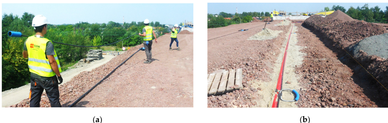
Figure 22. (a) The view of 3DSensor just before installation in the embankment; (b) the view of ready measurement line with 3DSensor and inclinometer casing.
